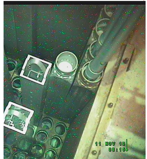
Photo taken during the November 2010 shut down
